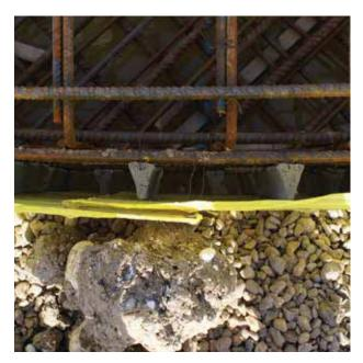
Heavy duty cementitious spacer bars have increased compressive strength and resist crushing
