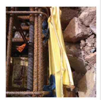
Spacer failure: Compressive strength exceeded by soil pressure, resulting in loss of cover
