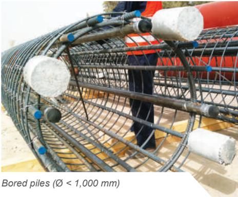
Bored piles ( $\varnothing < 1,000$  mm)
