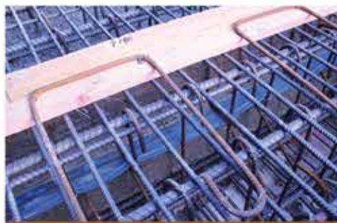
Construction joints at the Underpass using Stremaform
