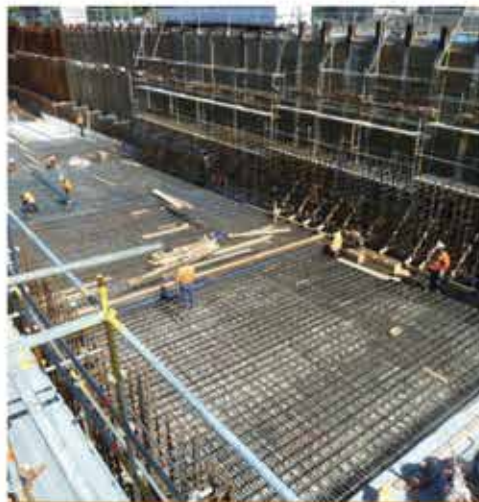
Memorial Park Underpass concrete slab in progress
